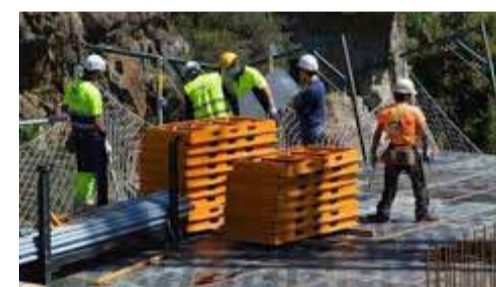
Workers on a construction site in the capital.
