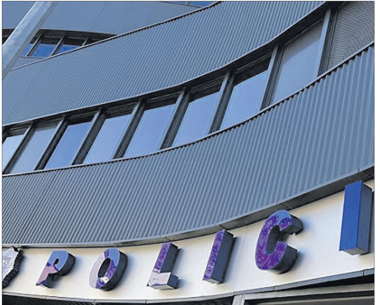
►► Police administrative building.
